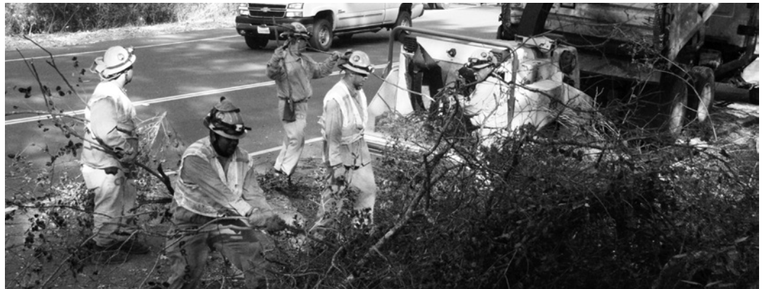
Road easement clearing.
