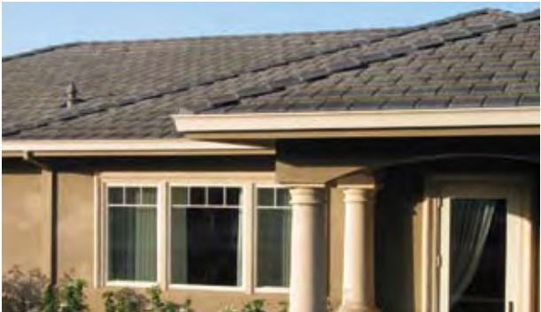
Fire-resistant roof, siding and double-pane windows
